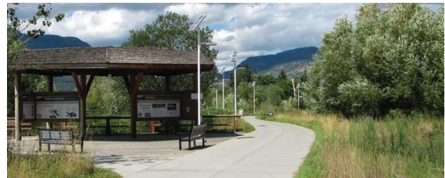
Example of solar powered pedestrian-scale lighting along path
