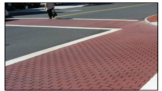
Example of Colorized Pavement
