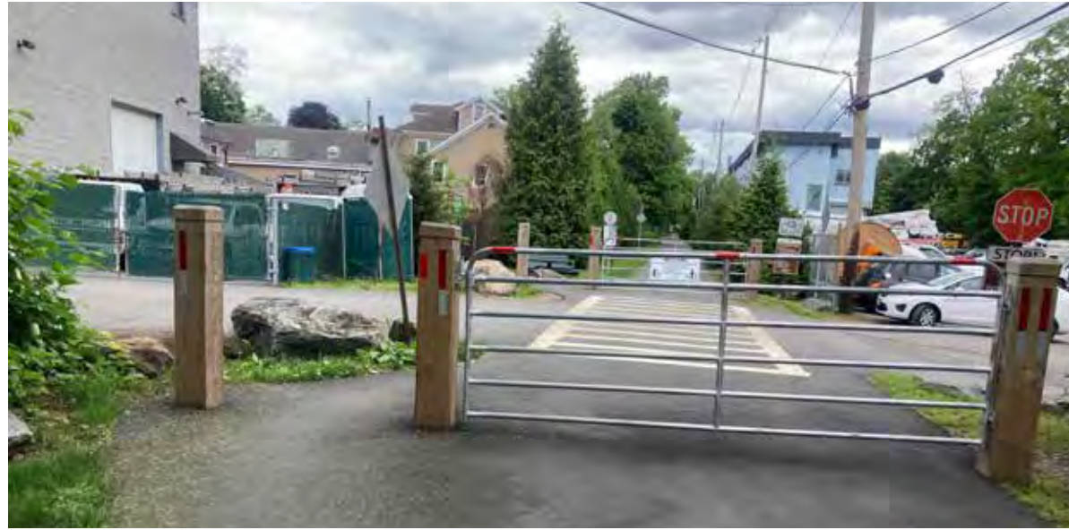
Gate for limiting motor vehicle use on trails while still providing emergency access
