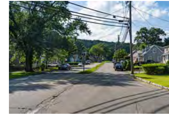
Existing conditions on Skyline Lakes Drive
