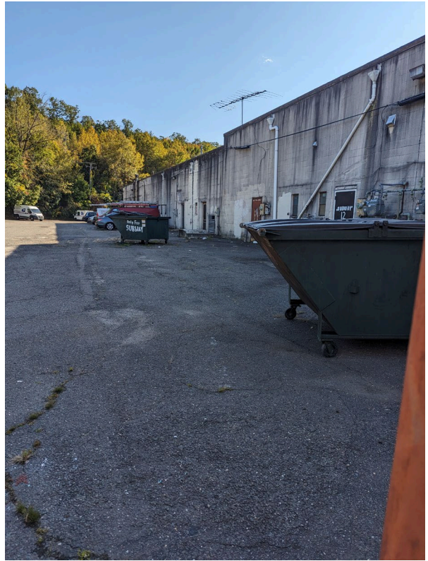
Photo 4 - Rear of shopping center, looking southwest
