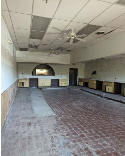
Photo 13 - Former cafe tenant space
