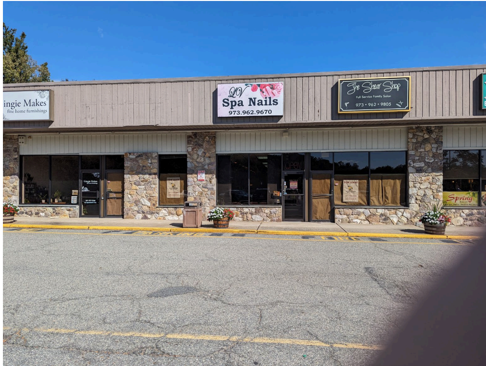
Photo 17 - Shopping center facade with two vacant tenant spaces visible
