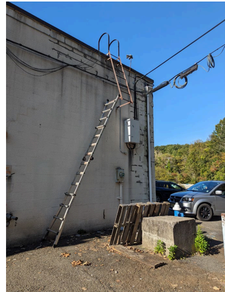
Photo 10 - Unobstructed roof access
